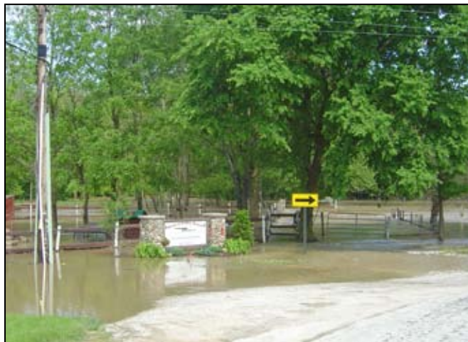
Natural Valley Ranch flooded driveway and fields
